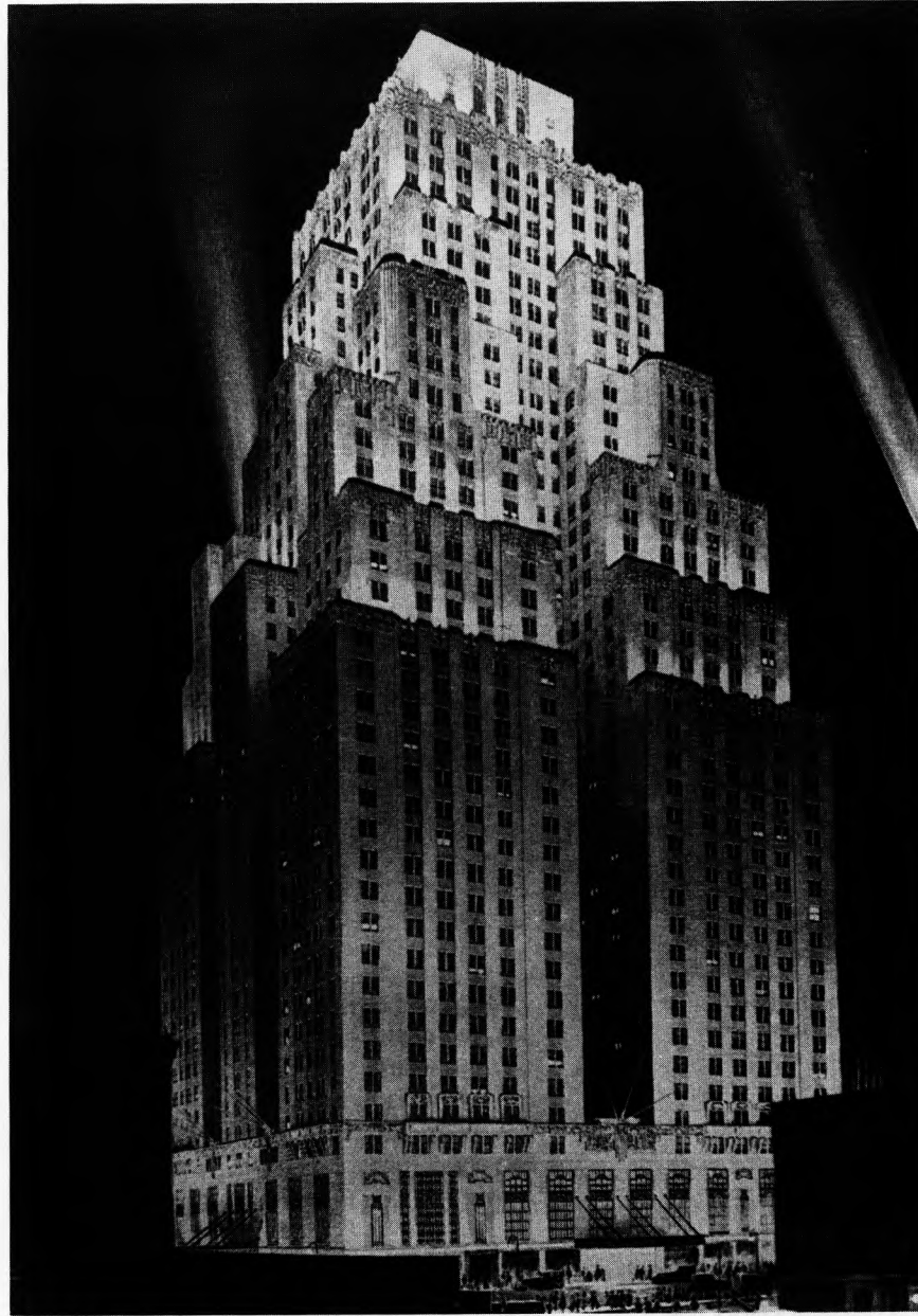
Figure 3.2 The New Yorker Hotel, completed in 1930, is a good example of "sculptured mountain" skyscraper architecture popular in the 1920s and 1930s, encouraged by the building setback requirements of New York City's zoning law. Urban planners, including the authors of the Regional Plan of New York and Its Environs , appreciated the setbacks and argued that high-rise structures should be situated farther away from surrounding buildings and streets than was mandated by the existing zoning. Source: Avery Architectural and Fine Arts Library, Columbia University.
